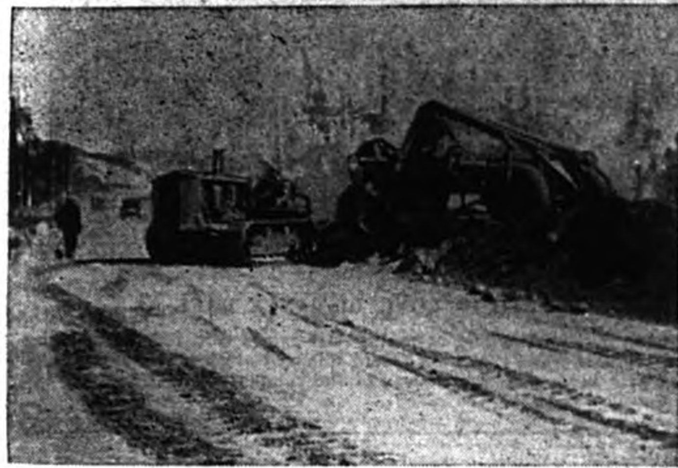
(Top) The Letourneau scraper, hauled by caterpillar tractor, makes the turn after dumping its load on the new grade.
