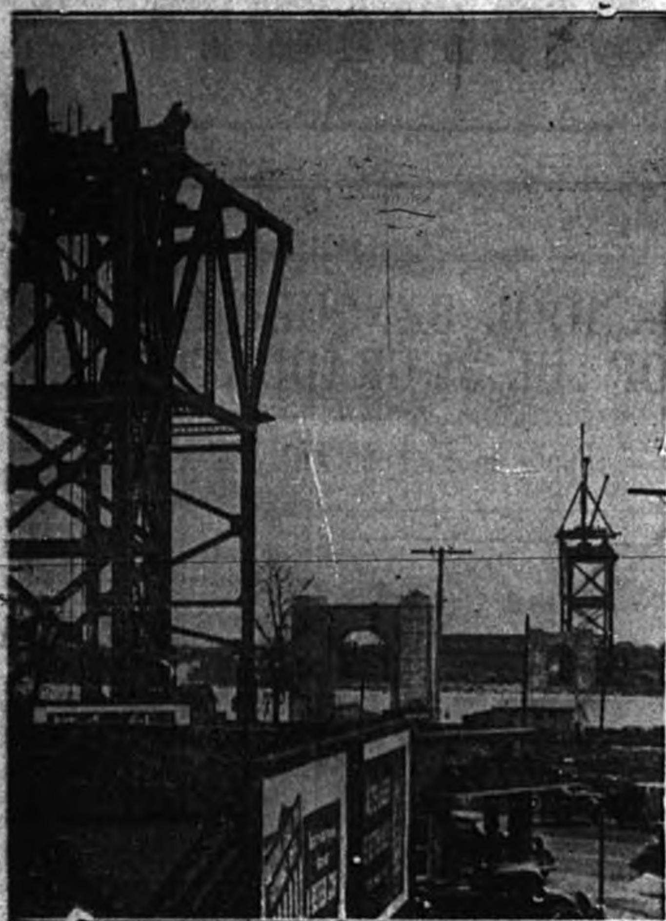
$3,000,000 BRIDGE BEING BUILT
