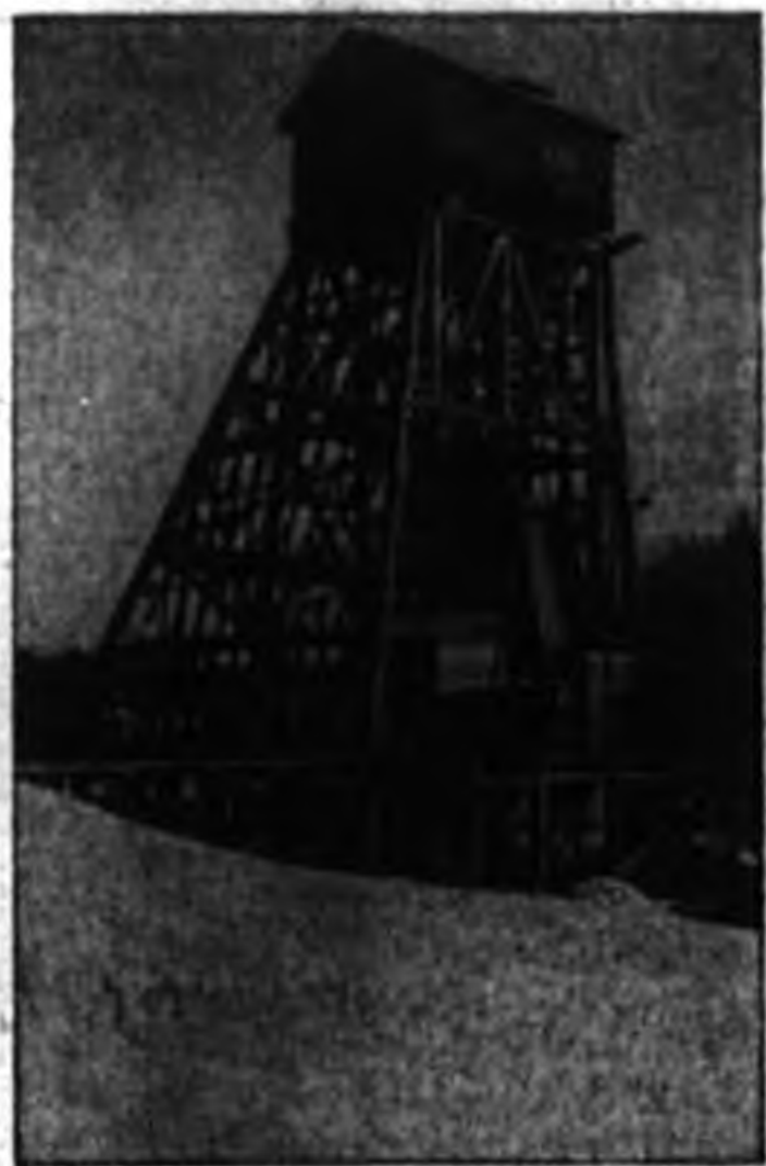
Mine headframe under construction.
