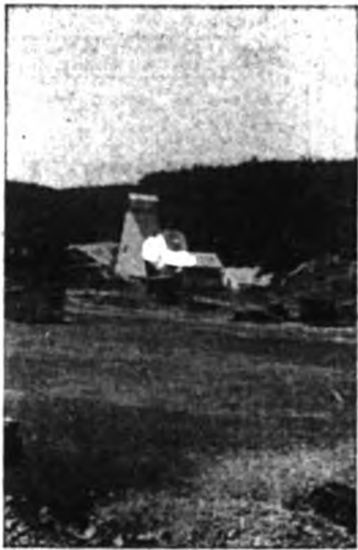
View of the mine buildings.
