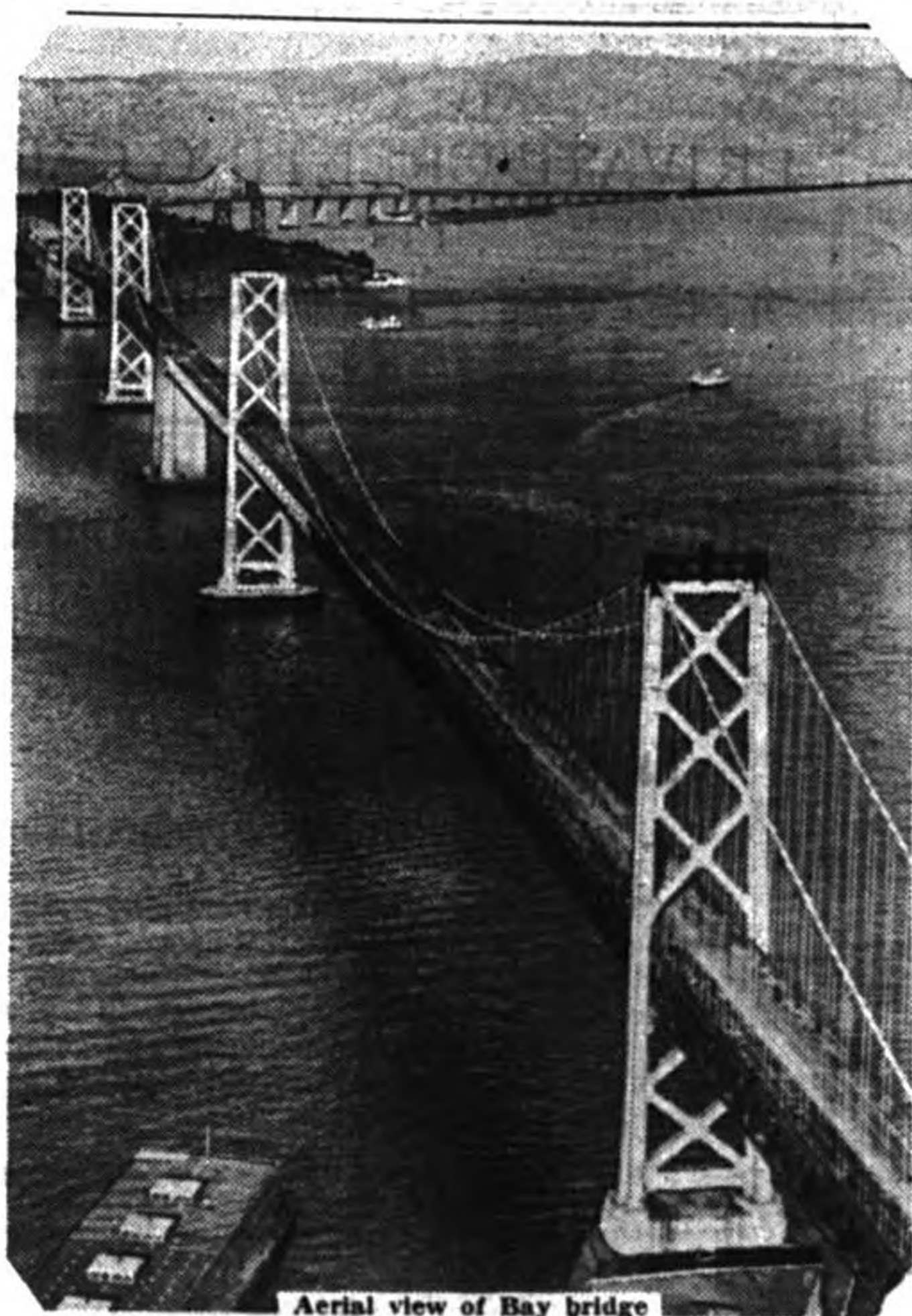
Aerial view of Bay bridge
