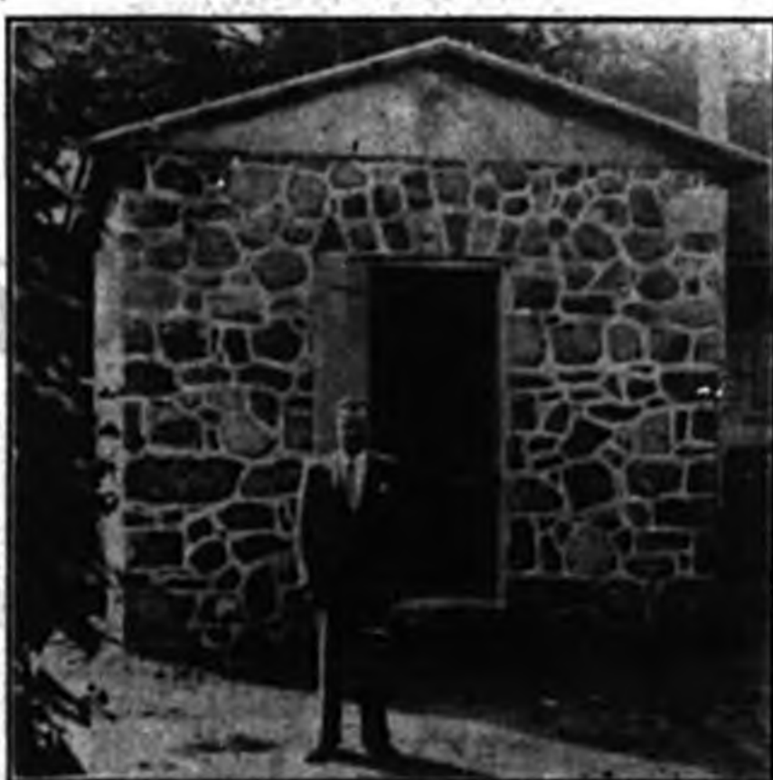
Oka Automatic telephone office with F. M. Dubreuil of the Bell Telephone Company (Montreal Suburban District, Sales)
