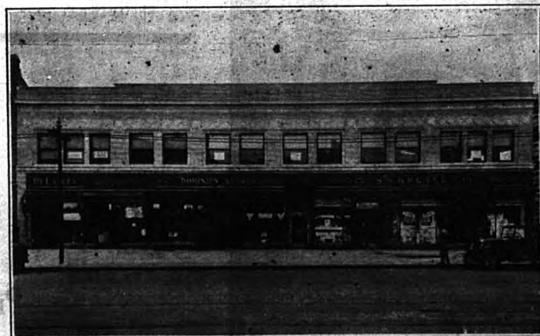
(Below) STORE BUILDING Corner Wilson Avenue & Sherbrooke Streets, Montreal. Erected for S. S. Kresge Company, Limited, by Richard & E. J. Ryan, Limited.
