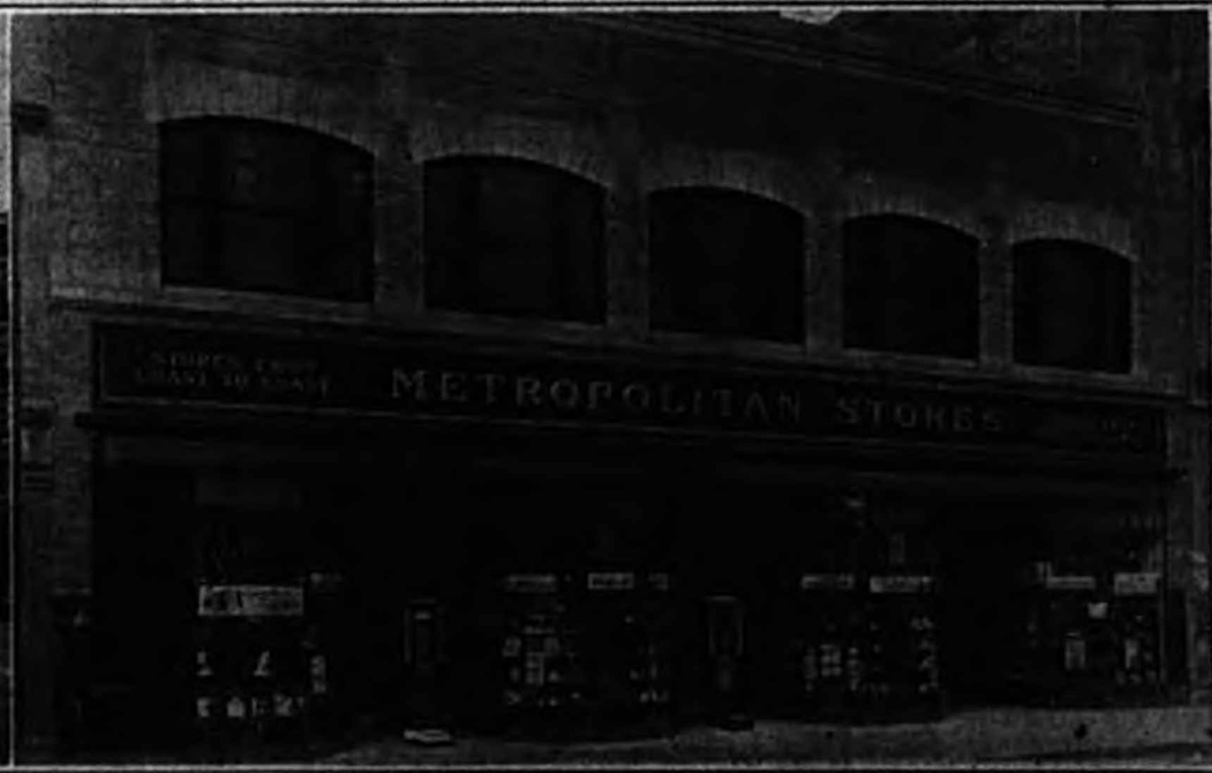
(Below) STORE BUILDING St. Joseph St., Quebec City. Erected for Metropolitan Stores, Limited, by Richard & E. J. Ryan, Limited.
