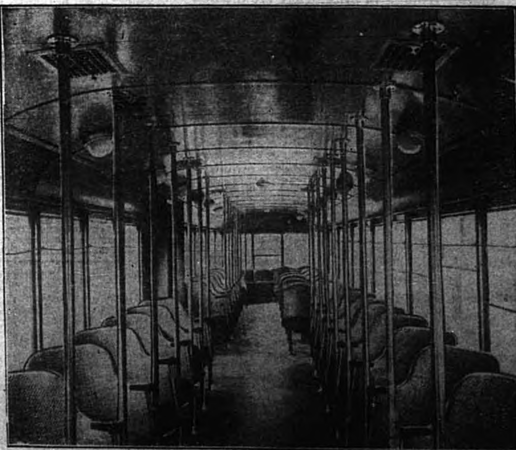
NON SKID COMPOSITION COVERS FLOORING IN ALUMINUM STREET CAR
