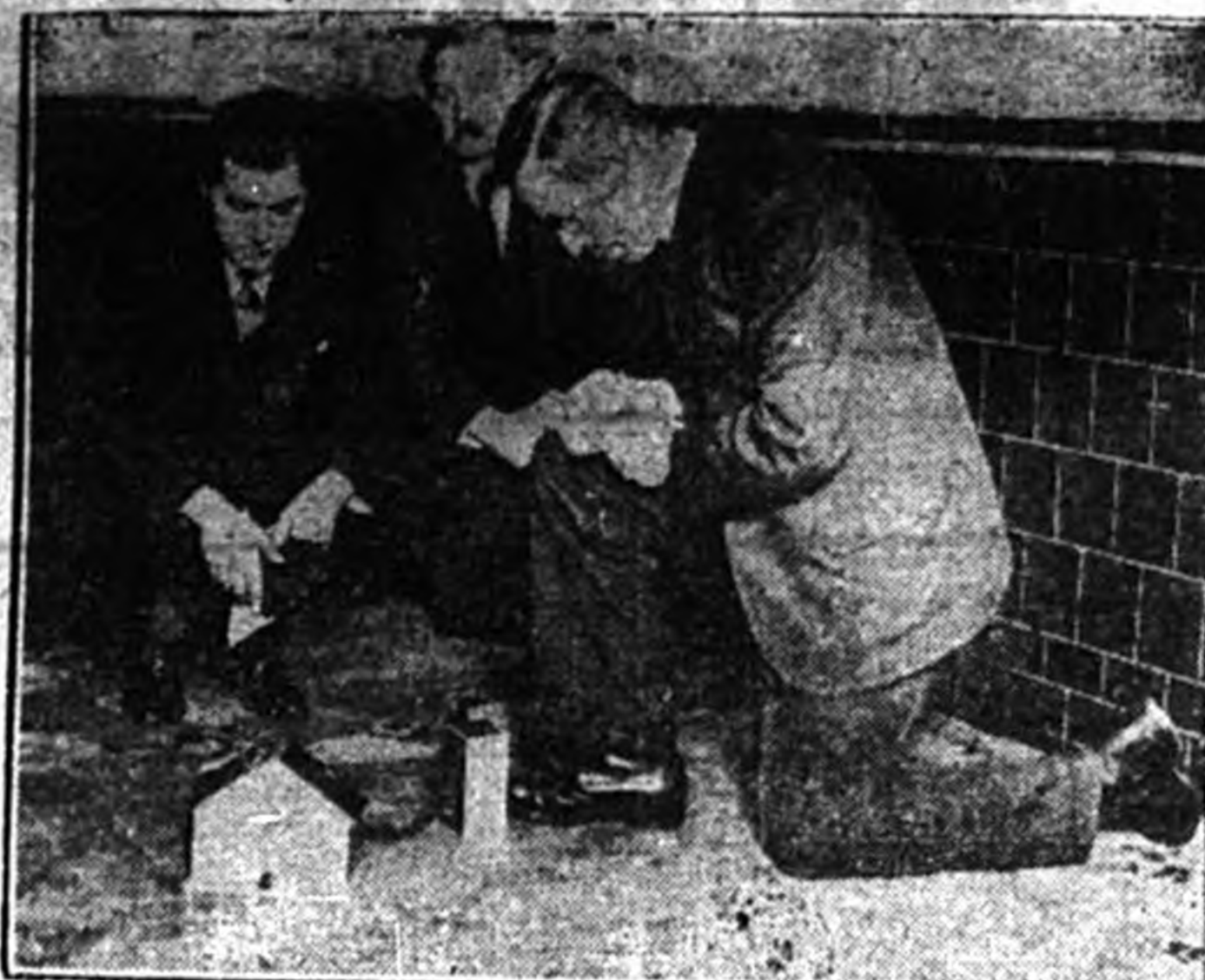
TESTING VIBRATORY EFFECT OF RUBBER ROAD
