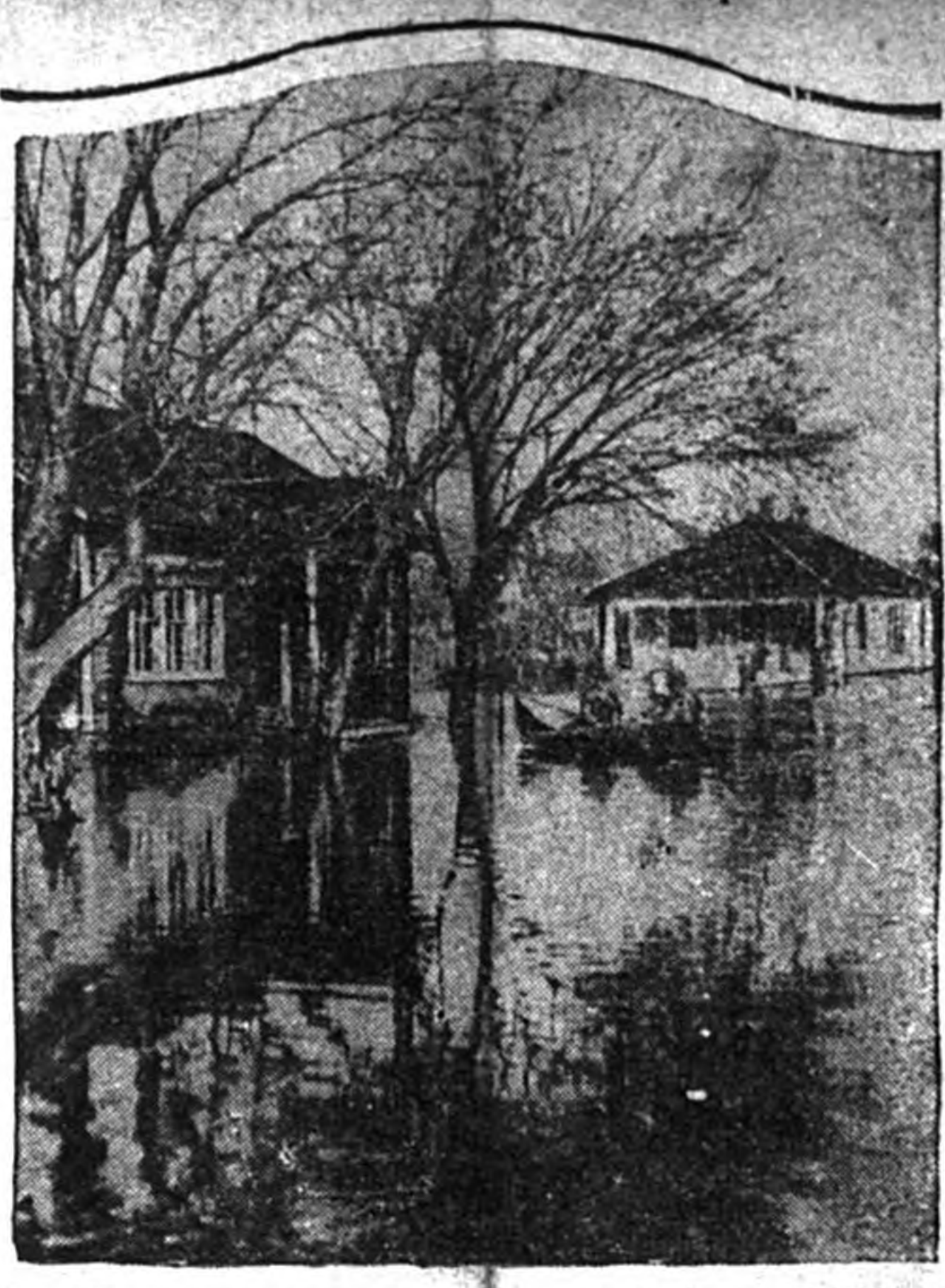
PROPERTY LOSS OF $10,000,000 CAUSED BY FLOOD
