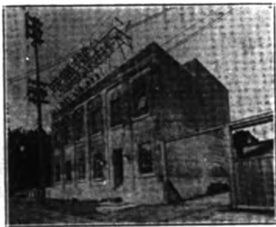
St. Jerome Substation
