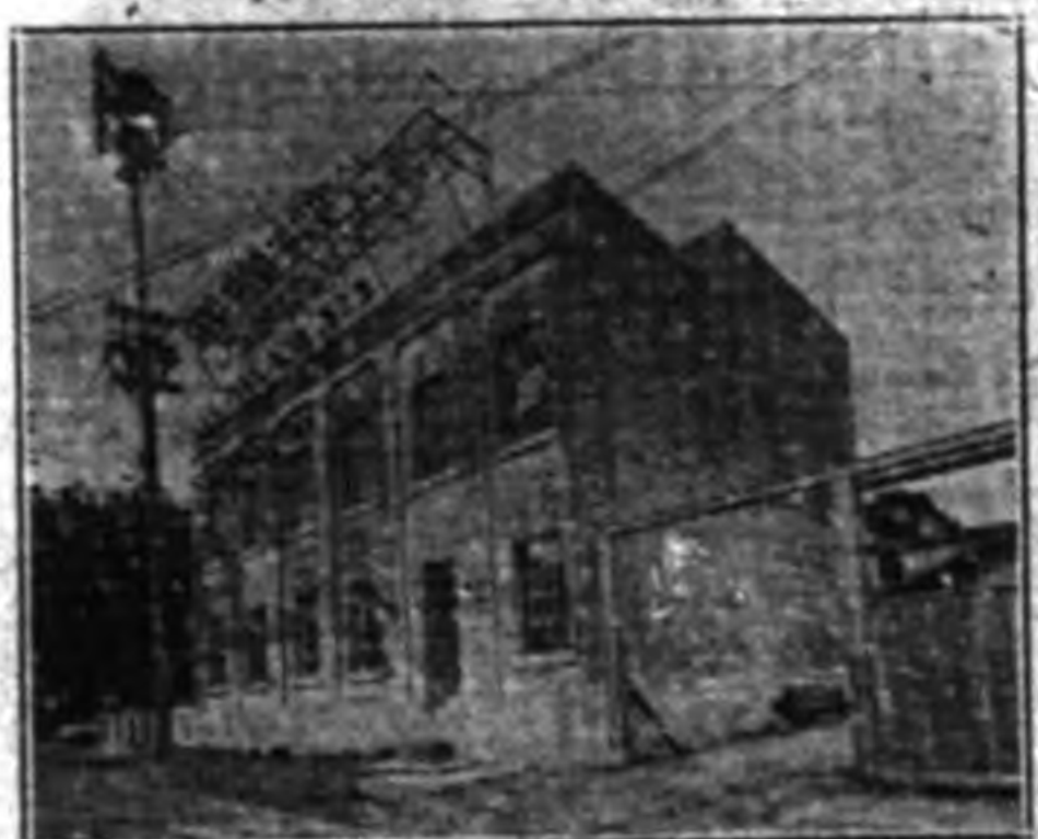
St. Jerome Substation
