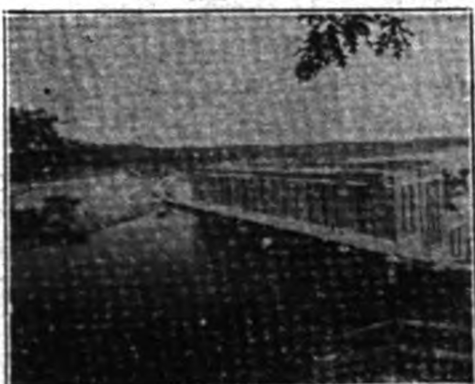
Exterior of Chelsea Power House
