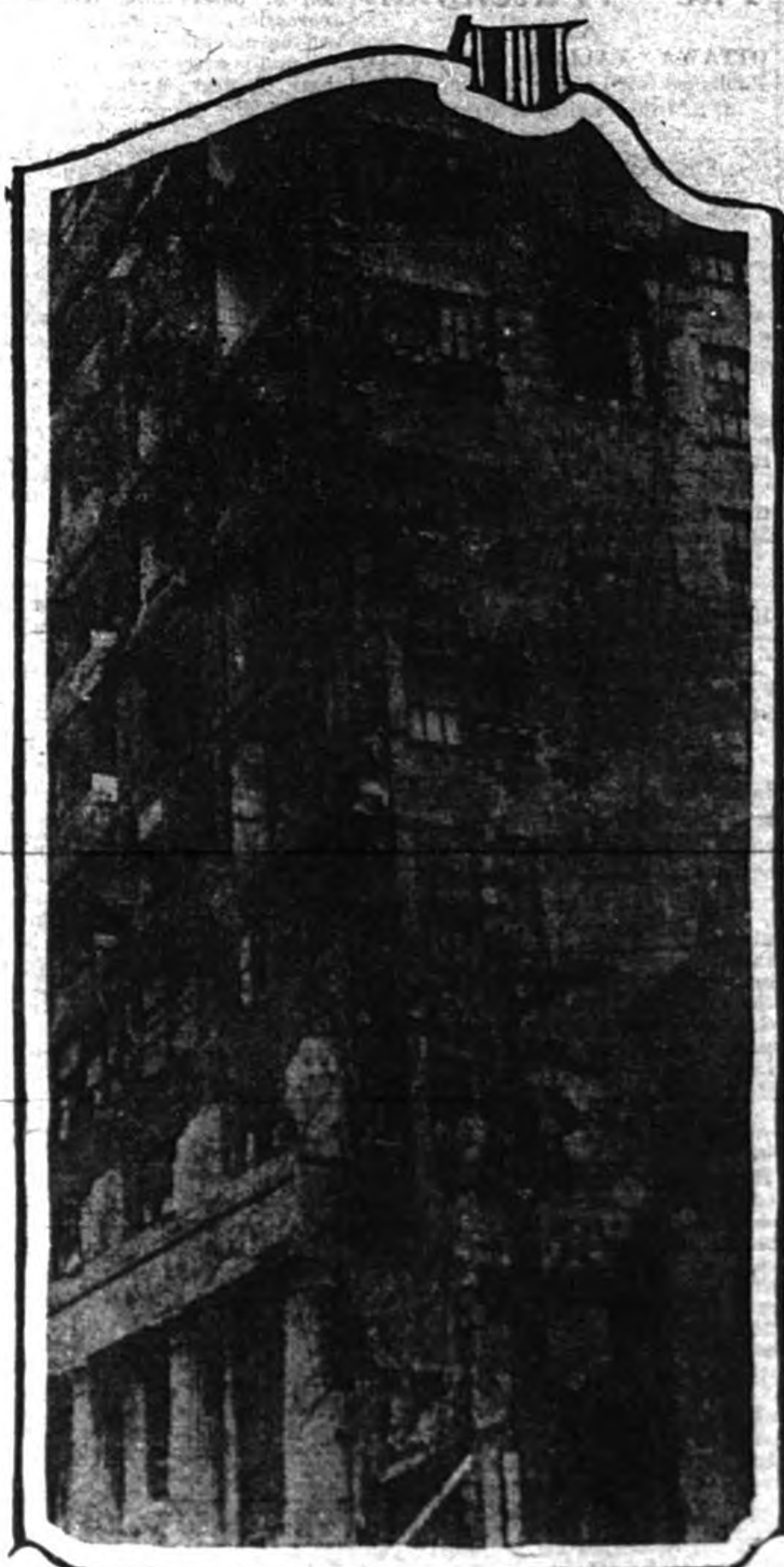
Ruins of the 14-story Meyer-Kiser Bank Building, Miami, Florida, which suffered severely from the hurricane of September 18th, and which will probably have to be completely torn down, are shown above.
