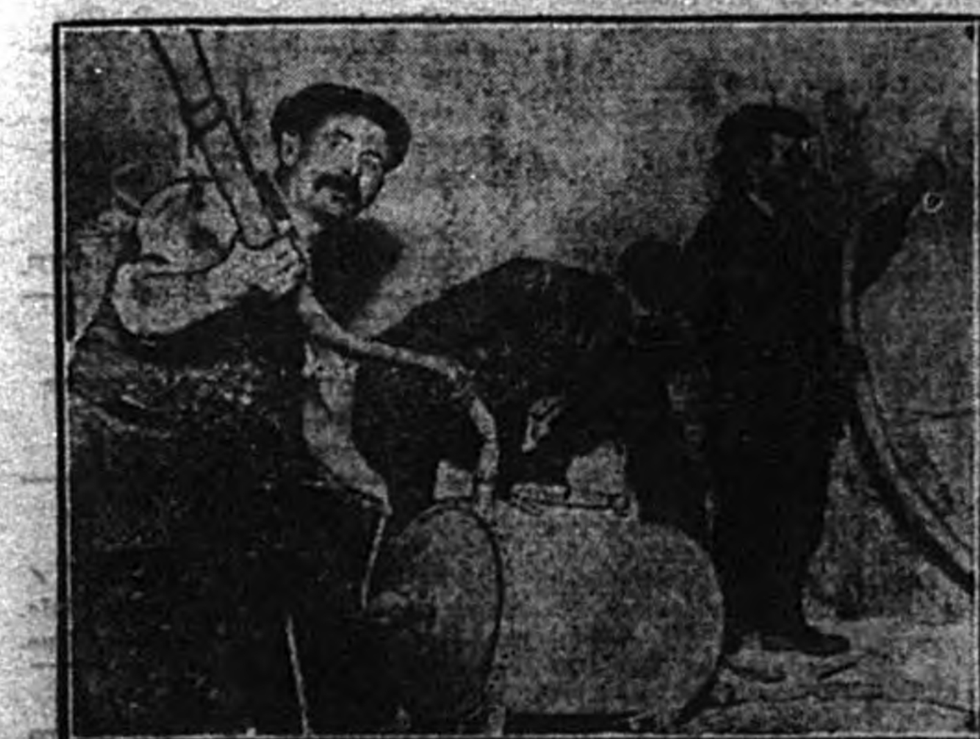
Workmen are filling the cracks in the dome of the famous St. Paul's Cathedral, London, with compressed cement, in their effort to save the towering edifice that has overlooked the city for so many years.
