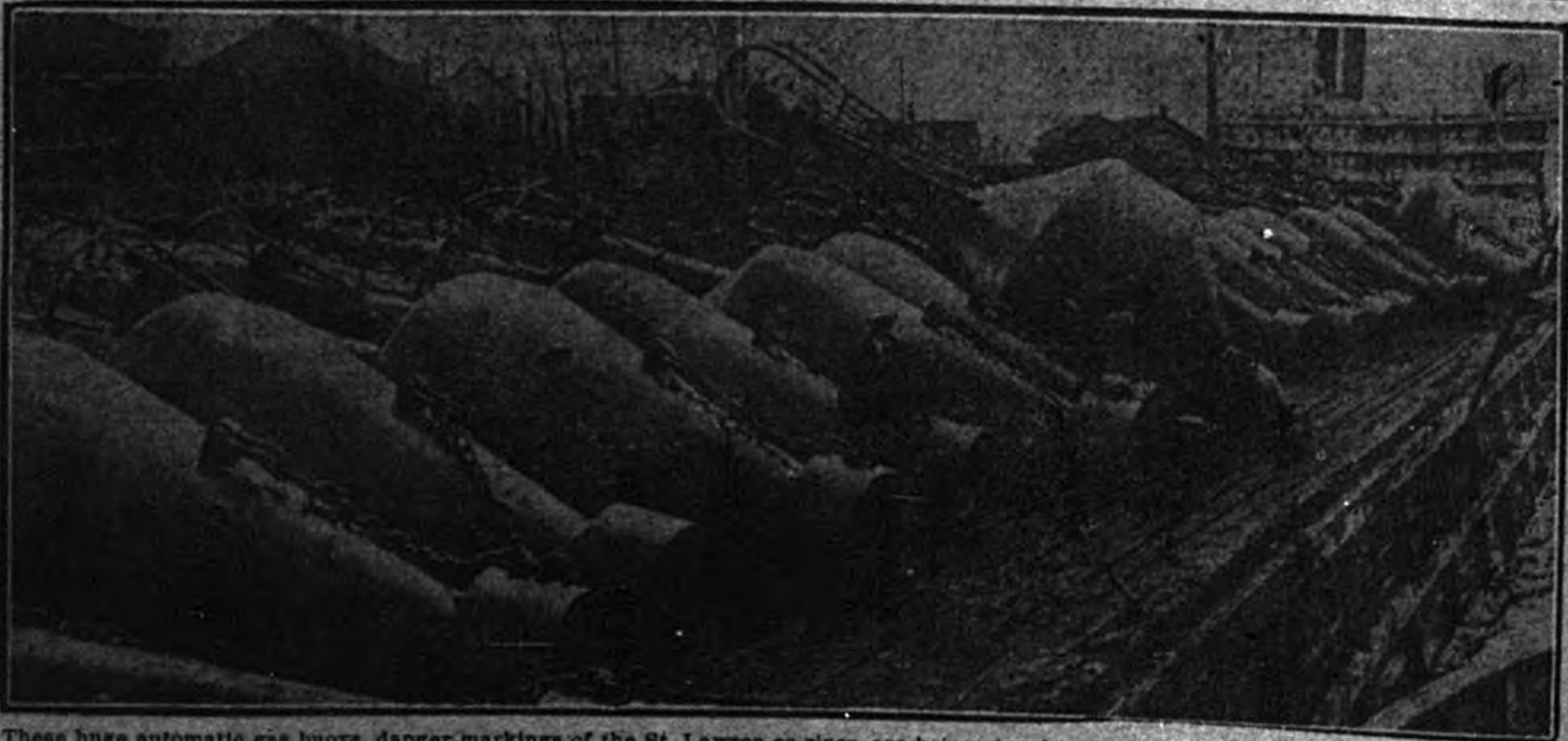
These huge automatic gas buoys, danger markings of the St. Lawrence river, are being stored away for the winter months at Sorrel, Quebec.
