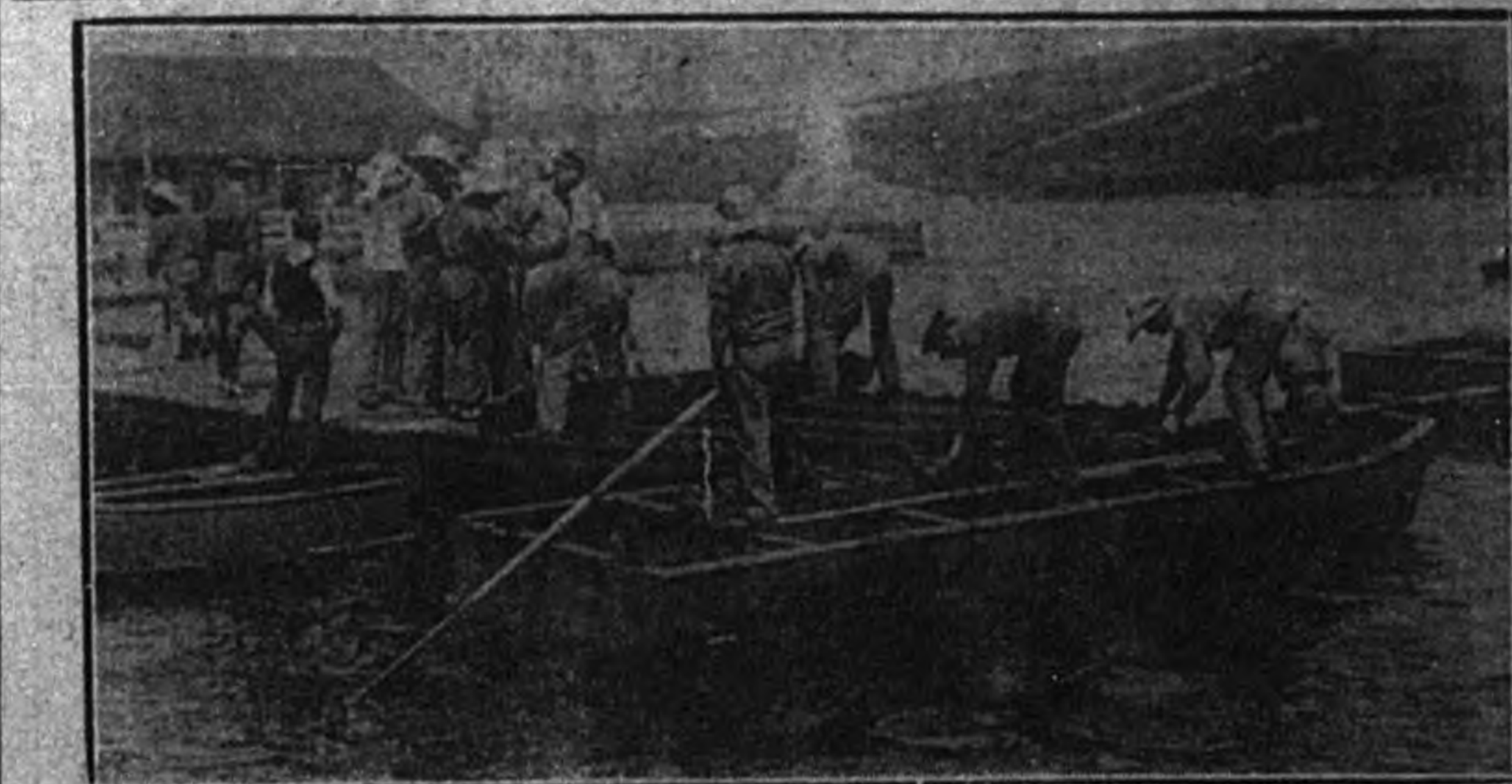
A detachment of Royal Canadian Engineers hauling pontoons together for the formation of a bridge in their recent field-day manoeuvres.
