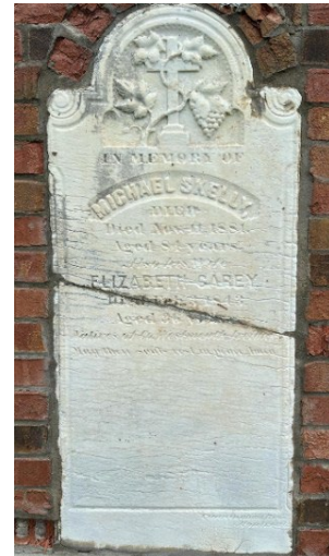
#12-Elizabeth Carey and Michael Skelly monument mounted on the wall and cleaned.
