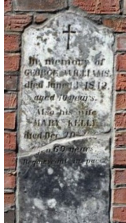
#155-George Williams monument mounted on the wall and before cleaning.
